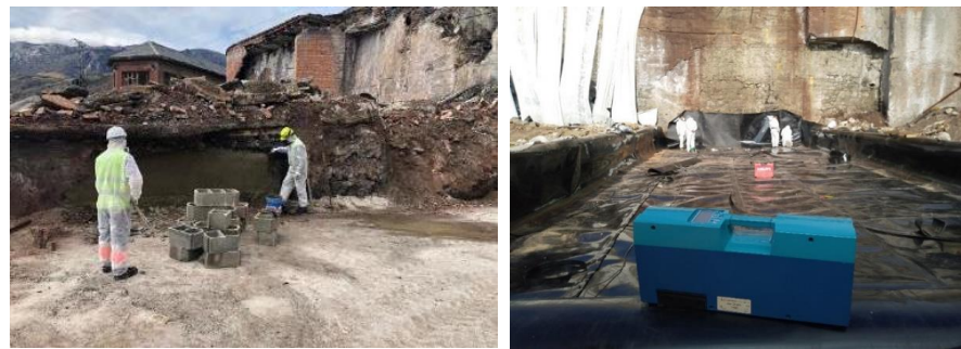
Figure 11. (Left): task 3 (perimeter wall construction); (Right): task 4 (HDPE sheet placement).
