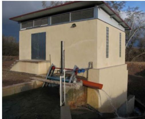
**Figure 3.** Water inlet to the loading chamber and side spillway.
