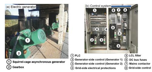
Figure 7. The different elements of the Barreda micro-hydropower plant.
